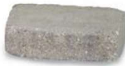
Weathered Cap Unit - B
